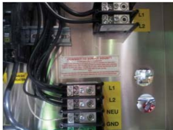
Main distribution blocks for connecting incoming single-phase
