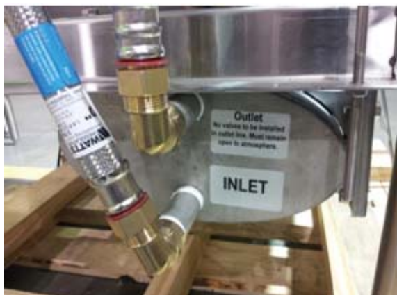
Flex hose connections (only hand tighten hose fittings)
