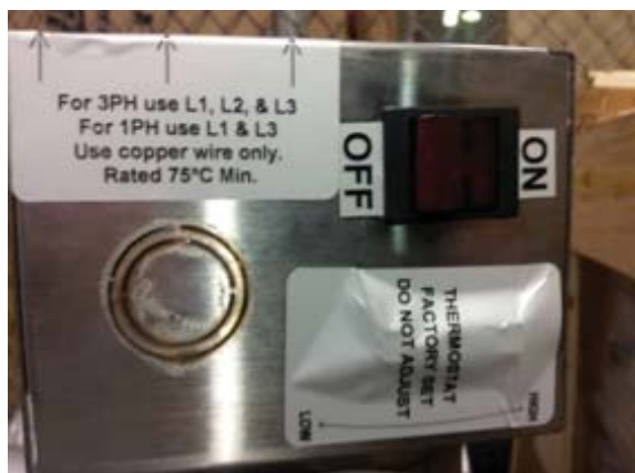
Pre-cut hole for conduit and power wires
