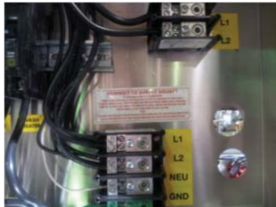
Main distribution blocks for connecting incoming single-phase
