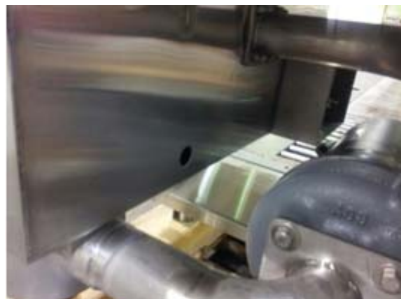
Showing 7/8" detergent probe hole behind pump motor
