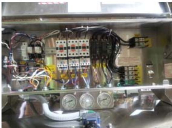
ADC-44 conveyor control box for single-phase power
