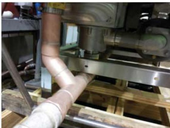
Showing 2" drain manifold exiting sump & scrap box
