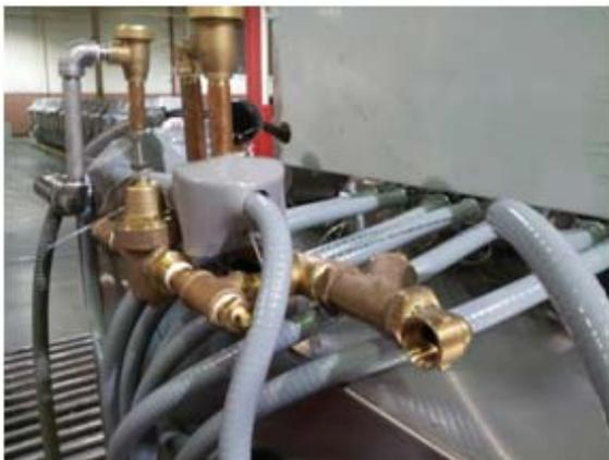
Hot water inlet manifold, single point ¾” pipe, PR valve
