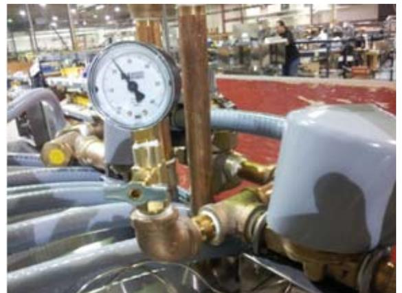
Final rinse manifold with pressure gauge, 20 psi flow req.
