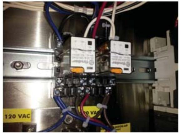
Conveyor motor control relays
