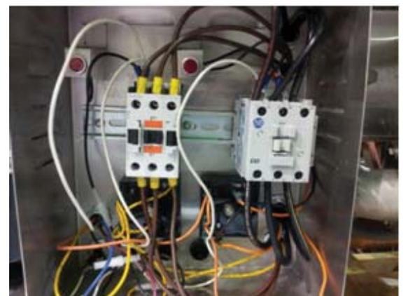
T-stat signal goes to term #6 on heater relay under contactor
