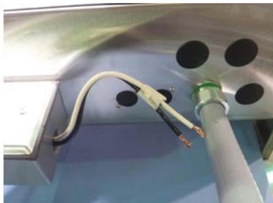
Showing power connection box for 120v wiring
