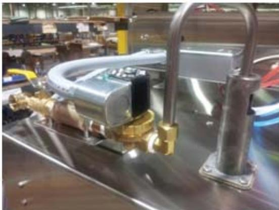
Showing 1/2" female pipe inlet, ball valve, y-line filter, water solenoid, ASSE approved air gap (backflow preventer)
