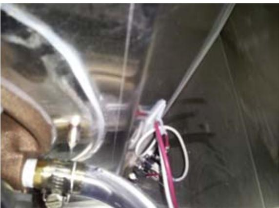
Heater terminals on right rear side of the tank
