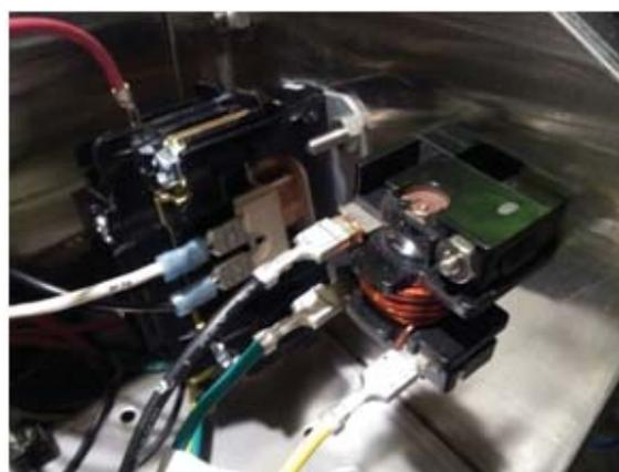
Wash motor contactor and motor relay
