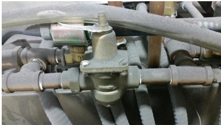
The union is seen at the right of the valve and has right hand threads with an o-ring seal
